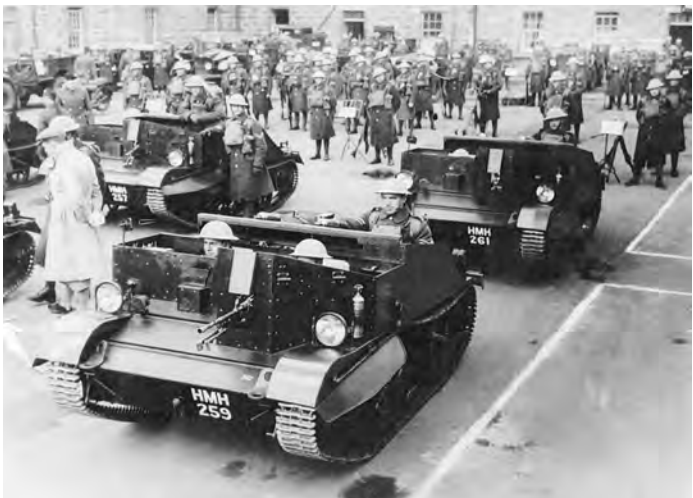
1939 (27 Mar). The Carrier Platoon carriers on the Mobilisation Parade. These light armoured and tracked vehicles had a good cross-country performance. Their armament was the Bren light machine gun, a magazine-fed .303" weapon slightly lighter and shorter in range than the GPMG (which is approximately the same calibre). The Carrier Platoon was a mobile machine-gun platoon. In the background can be seen two lots of rifles stacked or 'piled'. Above the upper sling swivel on an SMLE was the 'piling swivel'. These swivels were interlinked when the rifles were stacked ('piled').
