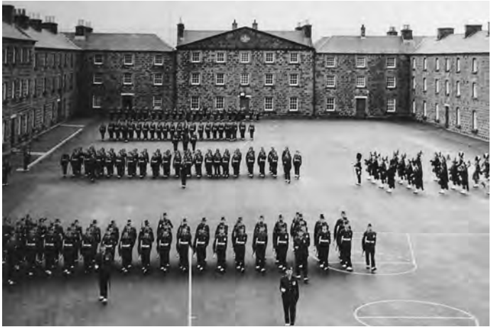
1967 (15 Dec). Annual Administrative Inspection; the March-Past. How many pipers on parade?
