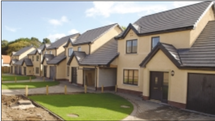
Some of the new Quarters at Glencorse.
